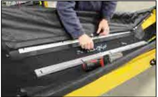
Fig 106 - Stainless steel hold-down bar to hold side flashing
