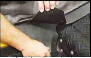
Fig 103 - Corner flashing against roller
