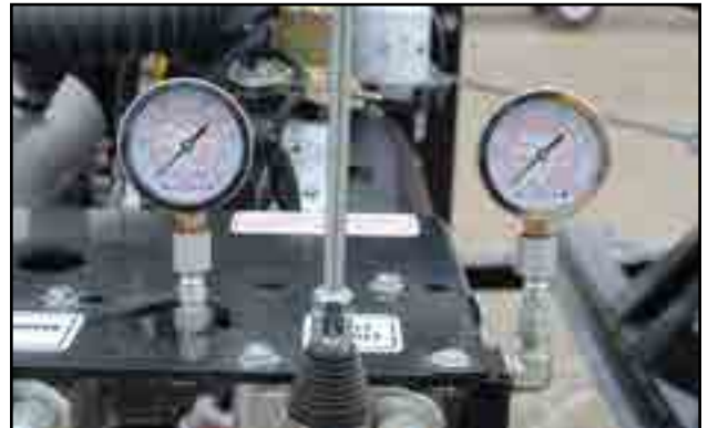
Fig 15 - Hydraulic pressure gauges
