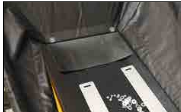
Fig 92 - Tail flashing on top of side flashing
