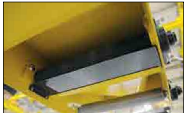
Fig 84 - Containment plate in place
