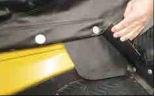
Fig 104 - Flashing fastened along transition
