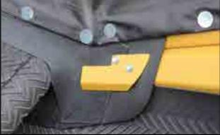
Fig 94 - Fasten flashing clamp
