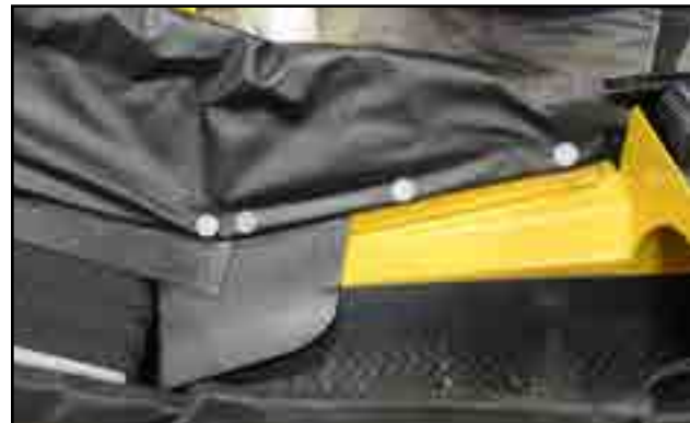
Fig 93 - Transition corner flashing in place
