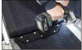
Fig 99 - Fasten transition flashing
