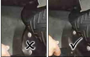
Fig 108 - Corner flashing must fit tight
