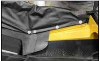
Fig 90 - Transition corner flashing in place
