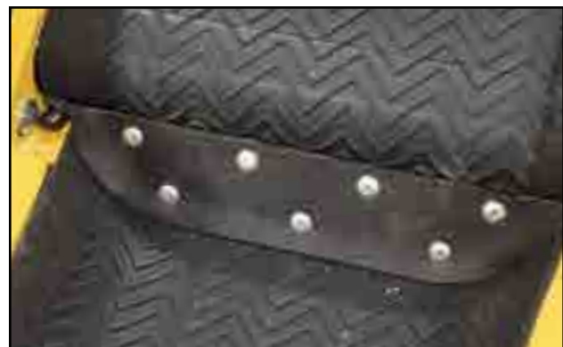
Fig 100 - Transition Flashing in place
